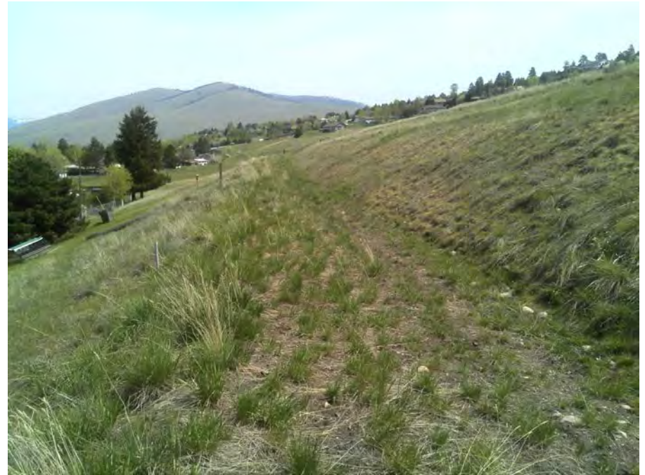
North center portion of site, note 8-foot high cut for drainage swale
