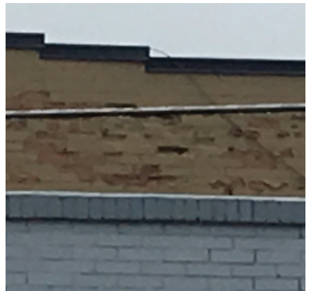
REPOINT DETERIORATING EXISTING BRICK -MATCH EXISTING
