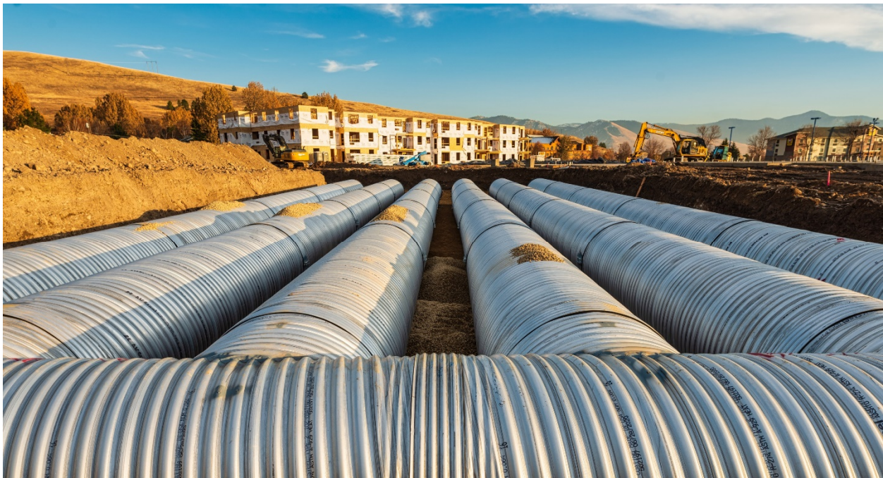
Figure 3. Underground detention storage installed for stormwater management.
