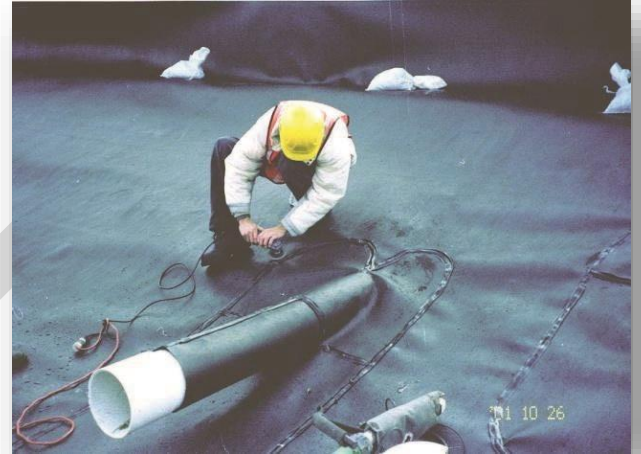
Technician seaming a 'boot' in a liner perforation. Photo credit: Panhandle Health District
