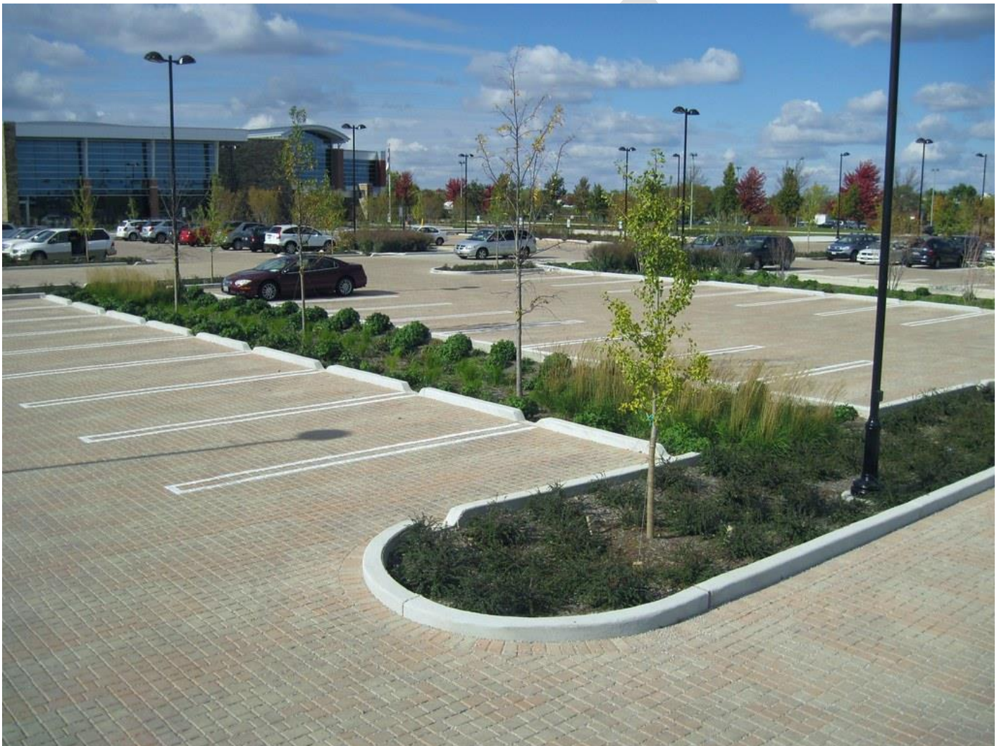
Parking lot bio swale design. "Conservation Design Forum Project: Fountain View Recreation Center, Carol Stream, IL" by Center for Neighborhood Technology is licensed with CC BY-SA 2.0. To view a copy of this license, visit https://creativecommons.org/licenses/by-sa/2.0/
