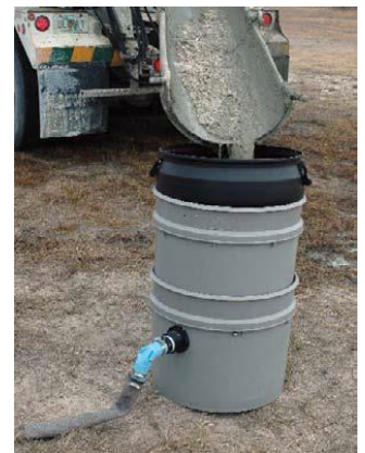
Filtering concrete washout water for reuse. Photo credit EPA.
