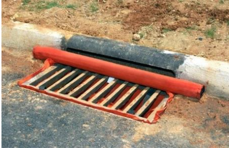
Dandy Sack placed within storm drain.
