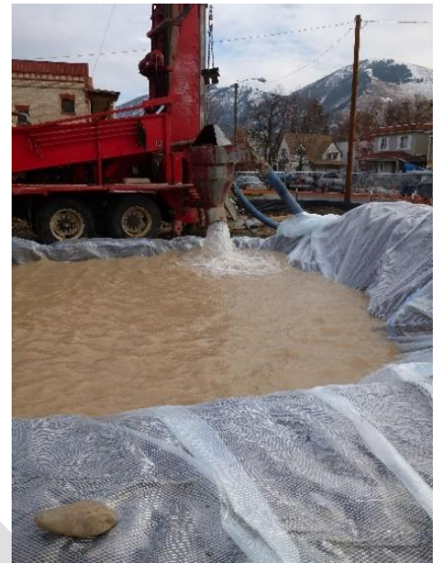
Sediment basin during well development. The rate of filling of this basin exceeded sedimentation. Filtration was necessary prior to discharge to the storm water system.
