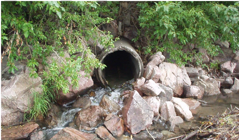
When rainwater enters the streets and alleys of Missoula, it can flow to nearby storm drains that discharge contaminated water directly to our local streams.
