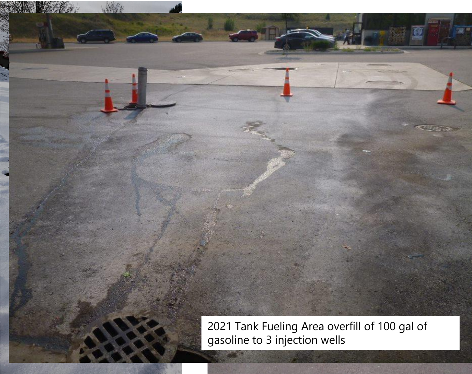
Drainage to injection well with evidence of past spill.
