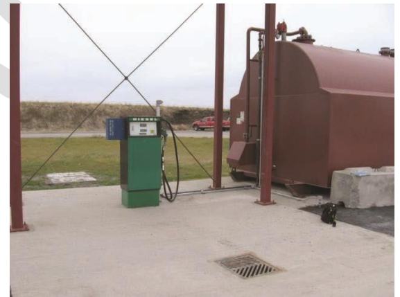
Private fueling site with triple-walled tank, catch basin, and separator (left background). Photo credit: Panhandle Health District
