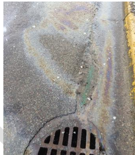
A good candidate drain for an oil-absorbent sock.
