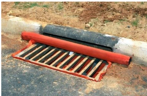
Dandy Sack placed within storm drain.
