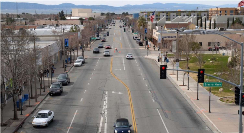
Figure 15: Lancaster Boulevard Before
