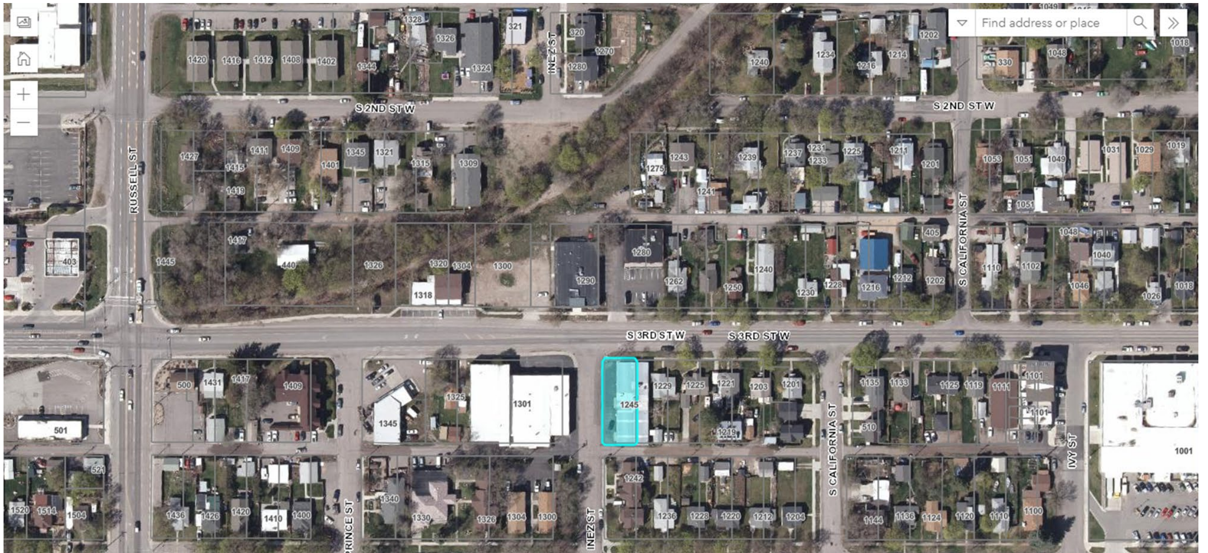
Project Location: 1245 S 3 rd St W – northwest corner of S 3 rd St W & S Inez St in URD II
