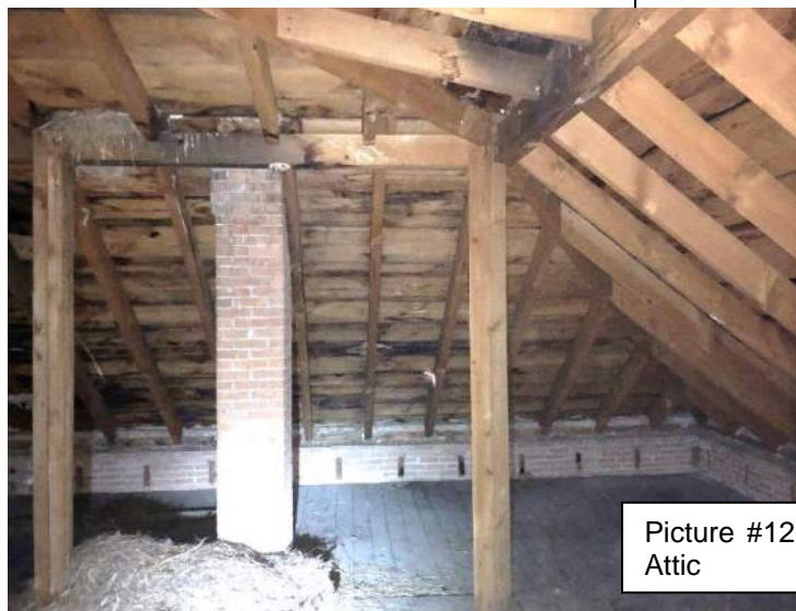
Picture #11 – Attic Girder/Posts & Rafters
