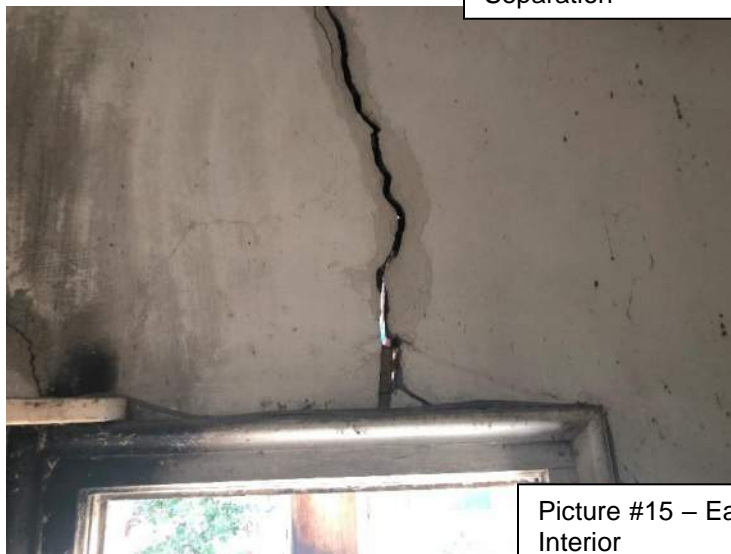
Picture #14 – East Wall Separation
