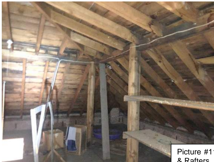
Picture #10 – Rafters Bearing on Exterior Brick Wall
