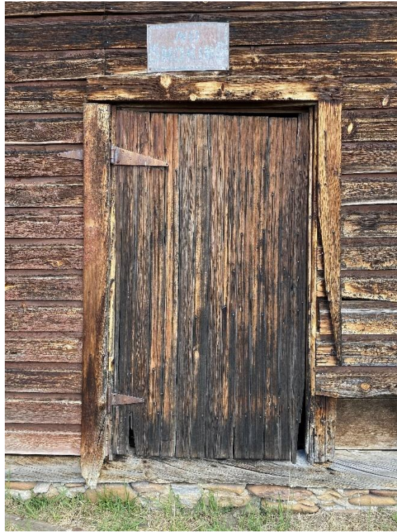
Figure 28. Photograph of representative door on the north elevation, showing door type, casement, and the uncut stone foundation.
