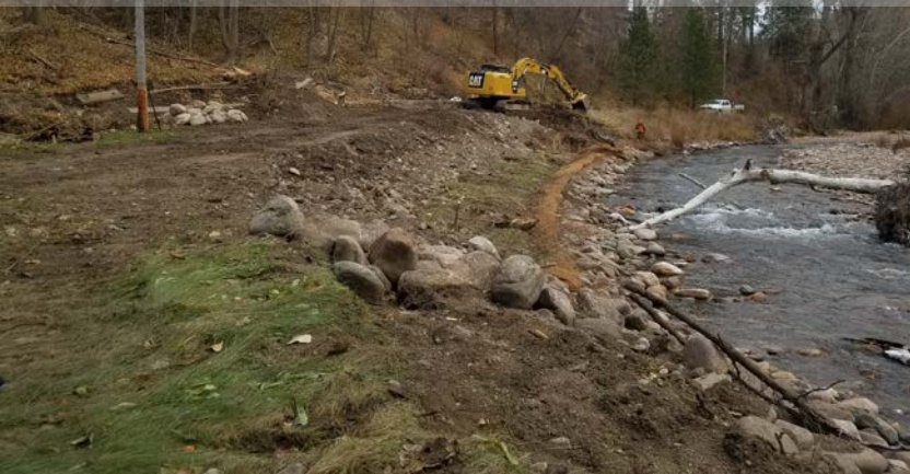
Bank stabilization, fixing a commuter trail & stormwater improvements in Greenough park
