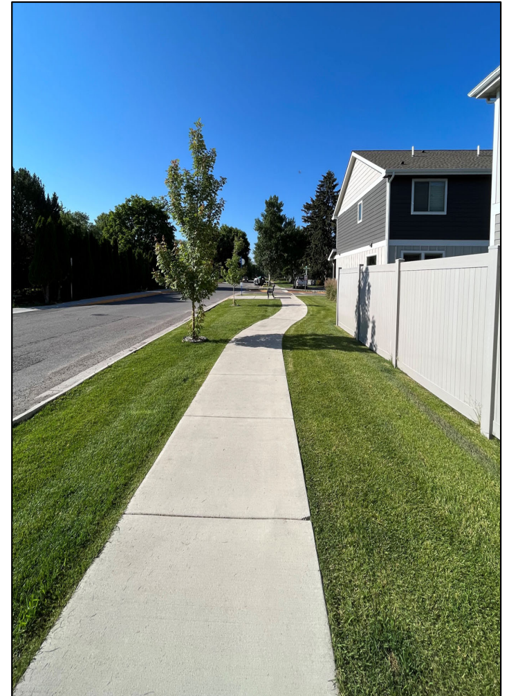
Eaton St. Phase 1 sidewalk and boulevard improvements
