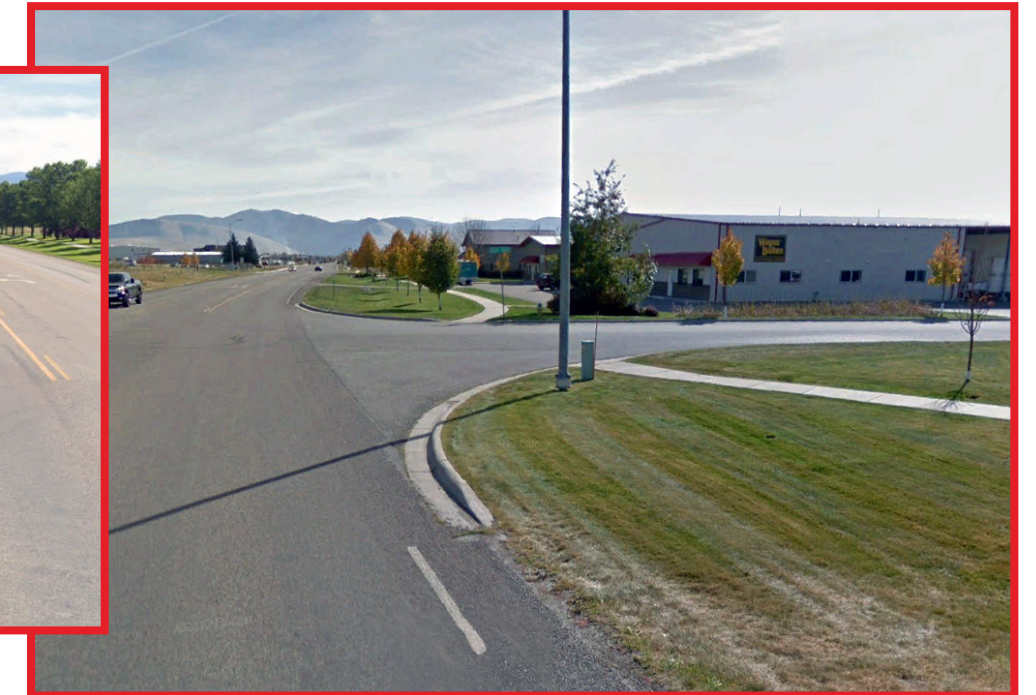
Wider curb cuts, separated multimodal facilities, and larger blocks support deliveries and large truck travel while providing for the safety of pedestrians.
