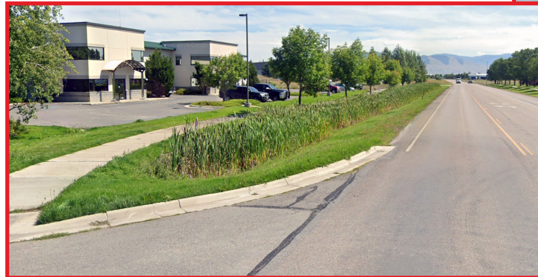
Effective stormwater management is necessary due to large areas of adjacent impermeable surfaces, as is typical with industrial land uses.
