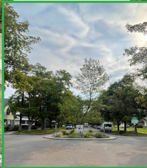
Frequent traffic calming limits vehicle traffic and speeds.
