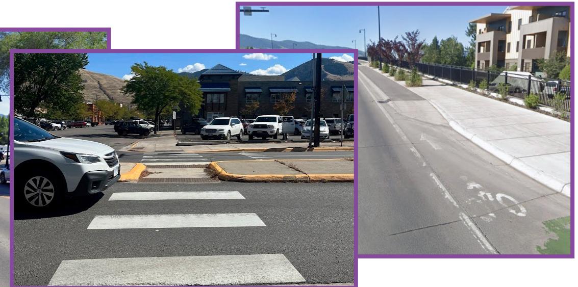
Short block lengths, frequent crossing opportunities, and pedestrian and bike facilities that are appropriate to network needs.
