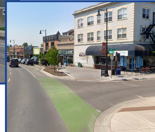
Protected bike facilities provide multimodal travel appropriate to the roadway conditions and network needs.
