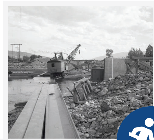
Russell Bridge Construction
