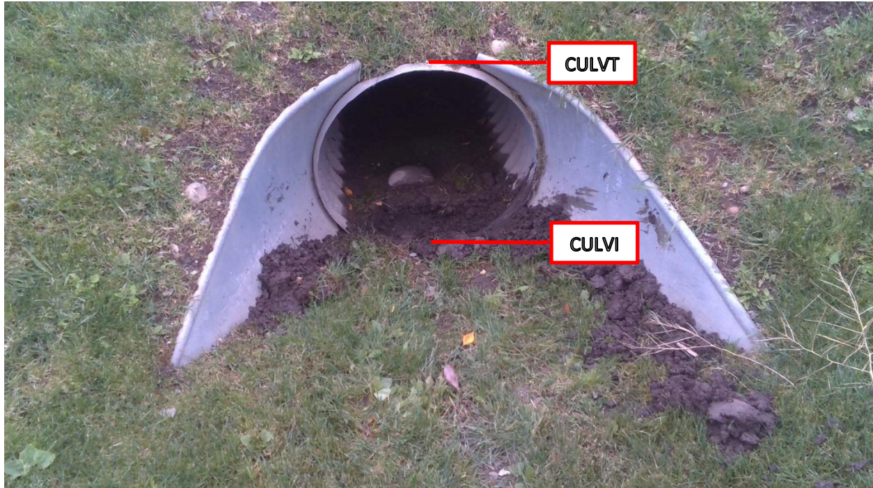
Culvert (with FETS)
