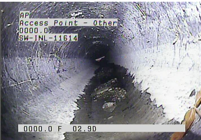
AP - Access Point - Other @ 0.0 ft. SW-INL-11614
