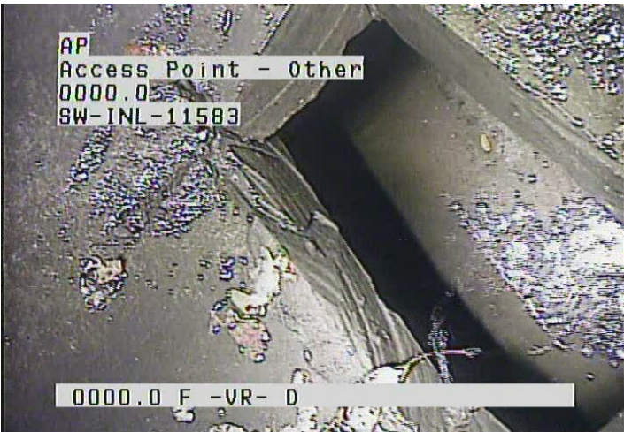
AP - Access Point - Other @ 0.0 ft. SW-INL-11583
