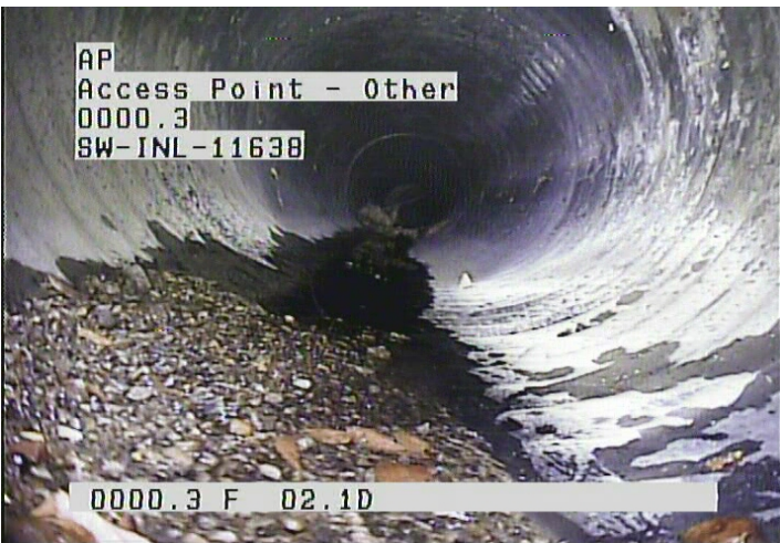
AP - Access Point - Other @ 0.3 ft. SW-INL-11638
