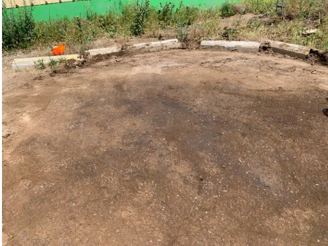
Asphalt pad discovered beneath the petroleum stained soil.
