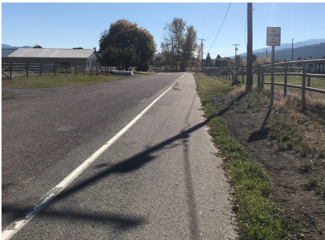
Widened shoulder as a designated walkway near Spurgin Rd
