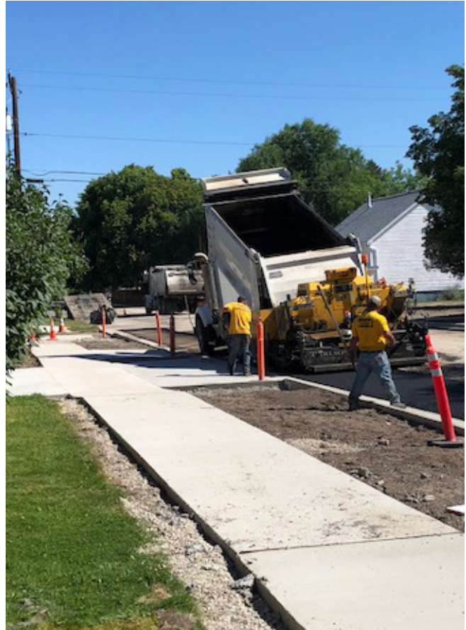
Construction of the Grant St Community Development Block Grant (CDBG) Project
