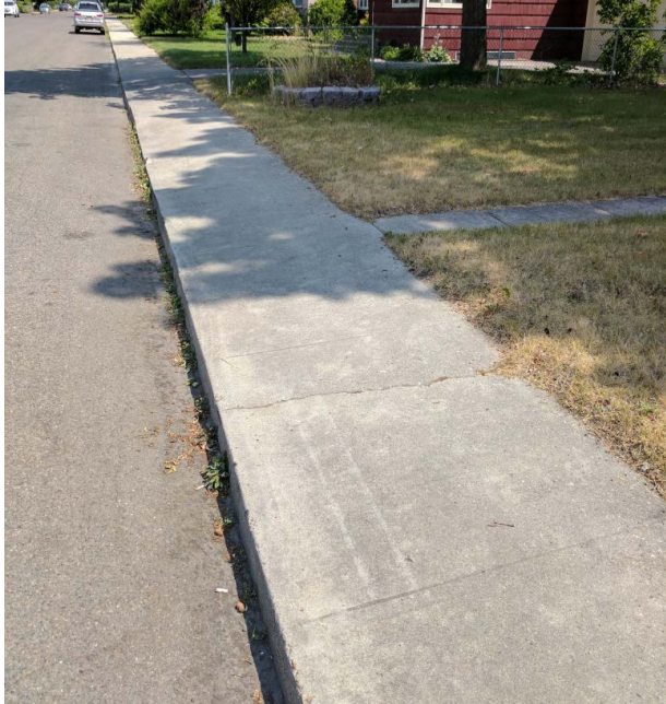
A-type combined sidewalk & curb (no gutter):
