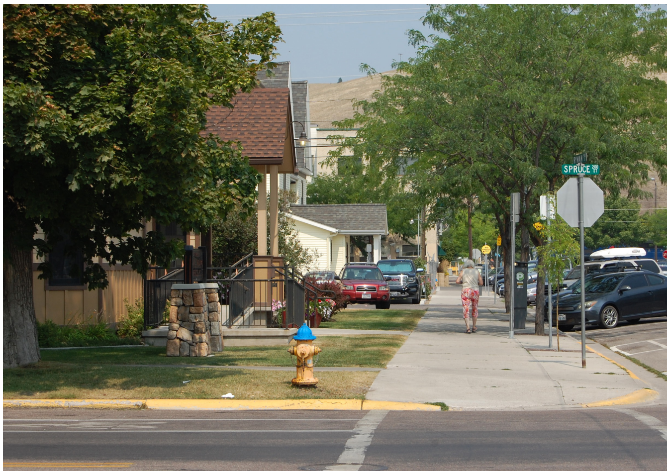
Non ADA-compliant pedestrian infrastructure along Spruce St
