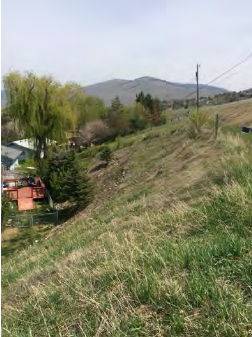
36-degree cut, 20 feet high near end of Saranac Drive
