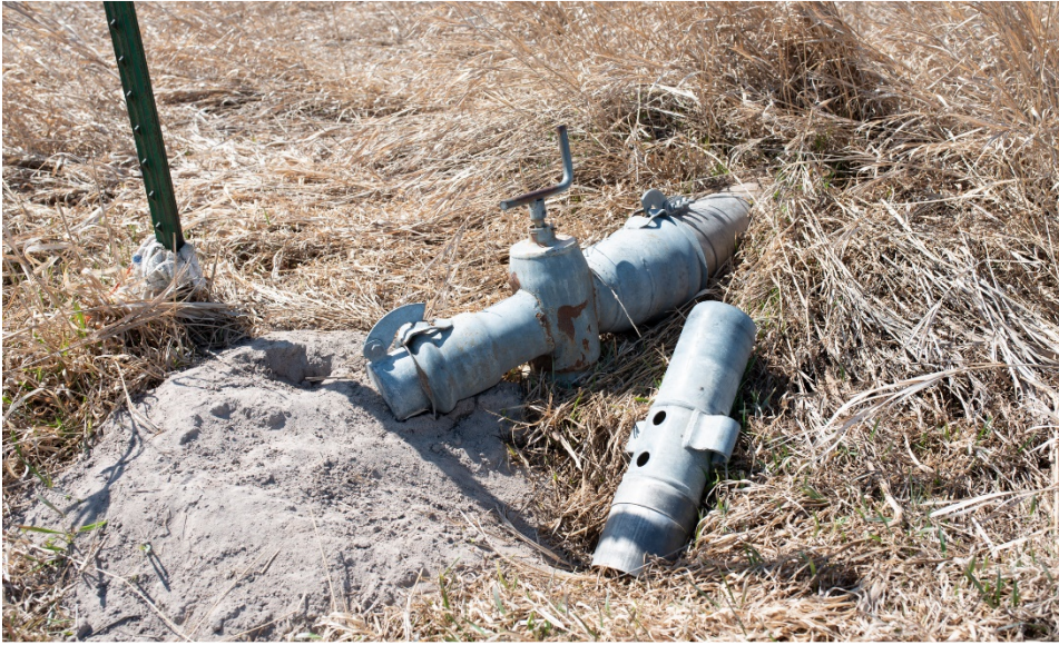
Figure 4. Connection between buried irrigation pipe and above-ground lateral pipe.
